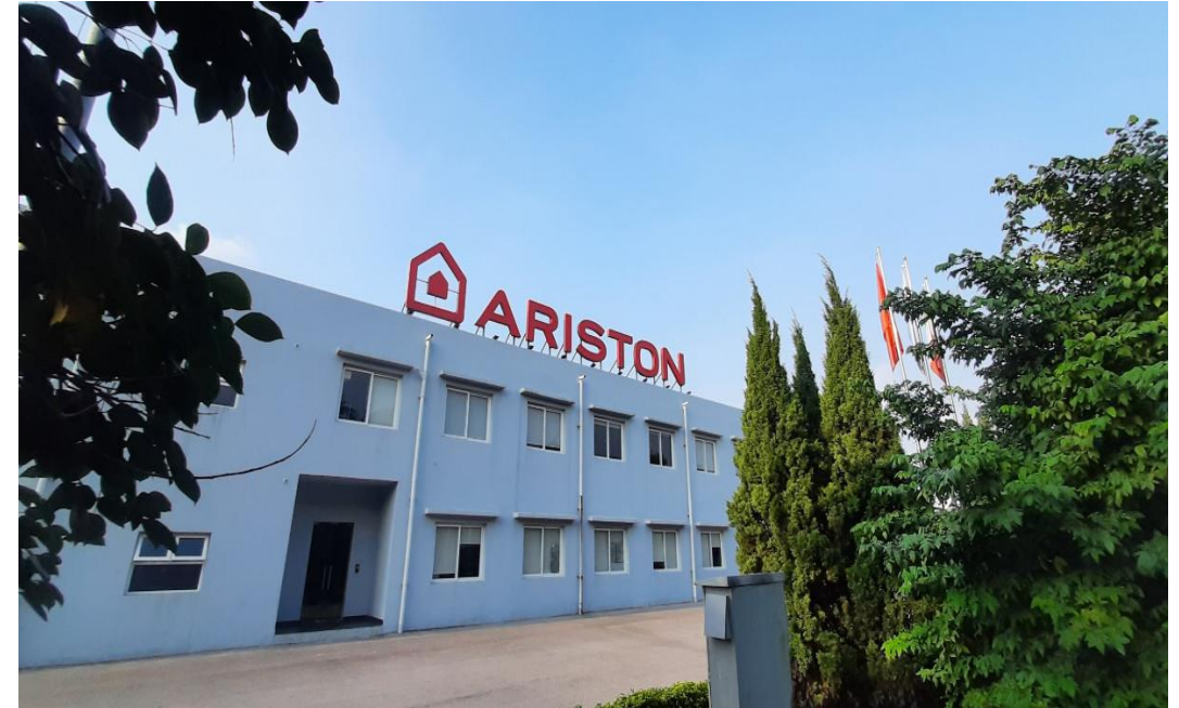
ARISTO FACTORY – BAC NINH (Vietnam)
