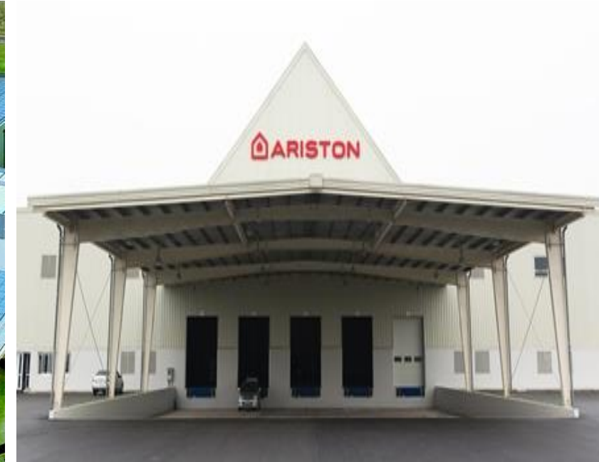
ARISTO FACTORY – BAC NINH (Vietnam)
